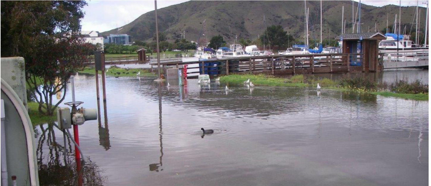
Figure 19. Oyster Point Marina Flooding During King Tide Event, 2021
