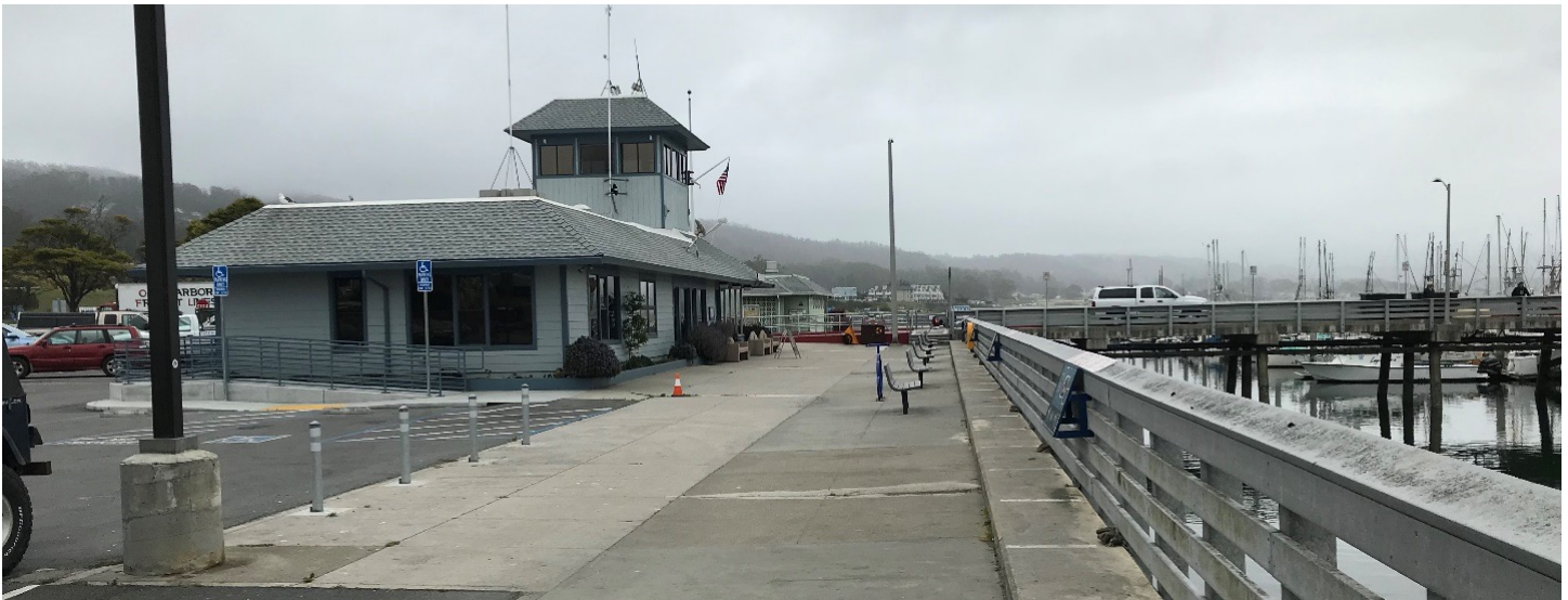
Figure 14. Pillar Point Harbor – Parking Lots, Buildings and Promenade, 2021
