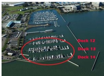
Oyster Point Marina Dock Replacement
