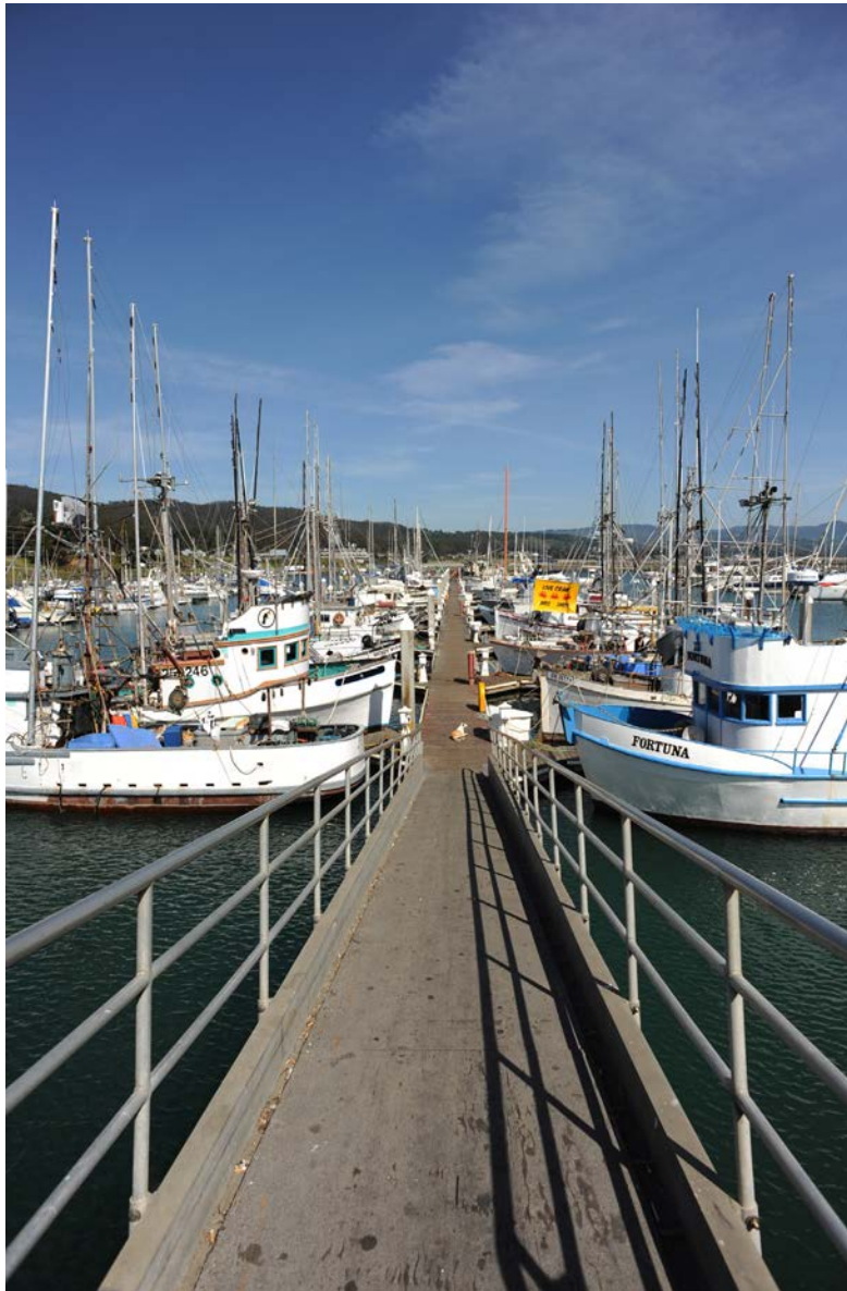
Photo: Finger Pier at Pillar Point Harbor
