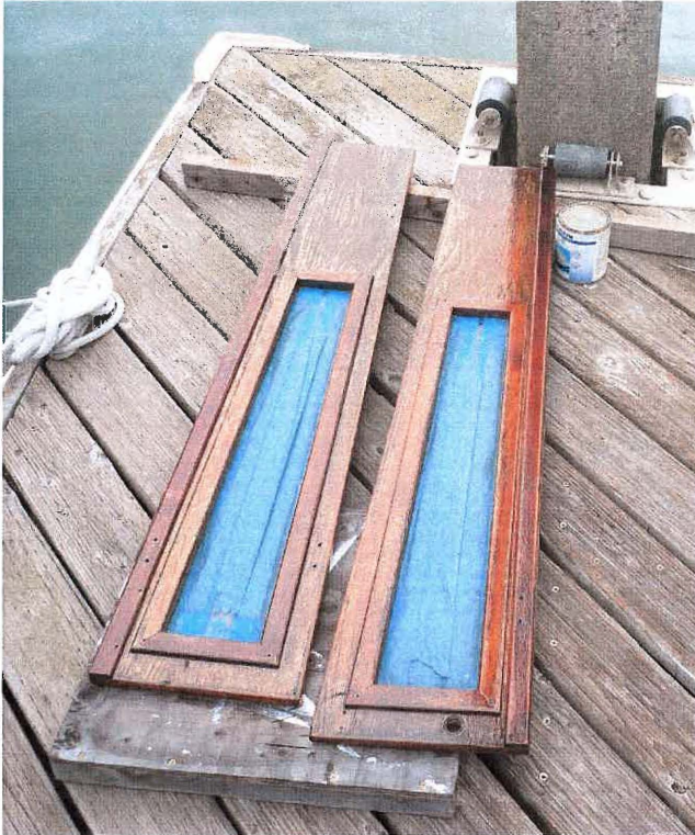
Photograph 21 Varnishing doors on the dock
