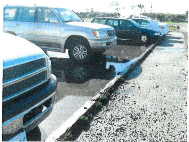
Photograph 11: Paved Parking Lot
