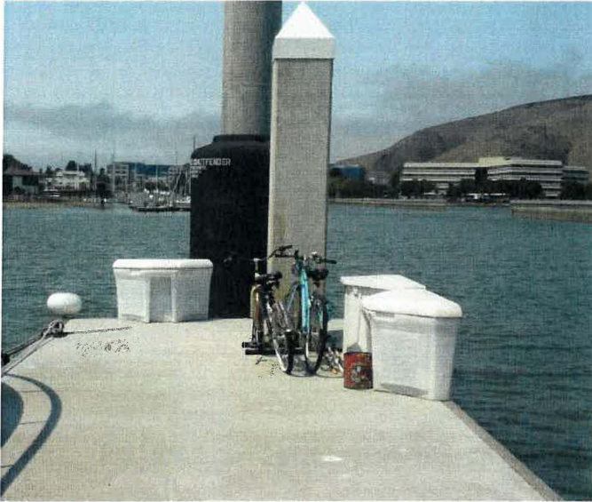
Photograph 18 Bike rack, bicycles, and tenant installed dock boxes
