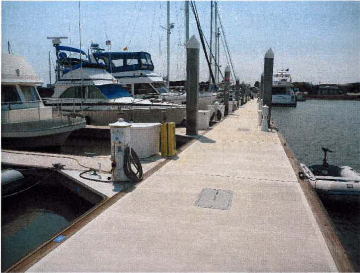
Photograph 2 General appearance of Dock 11
