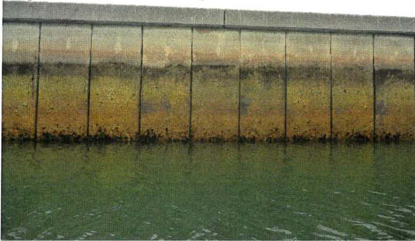
Photograph 26 Section of breakwater in good condition
