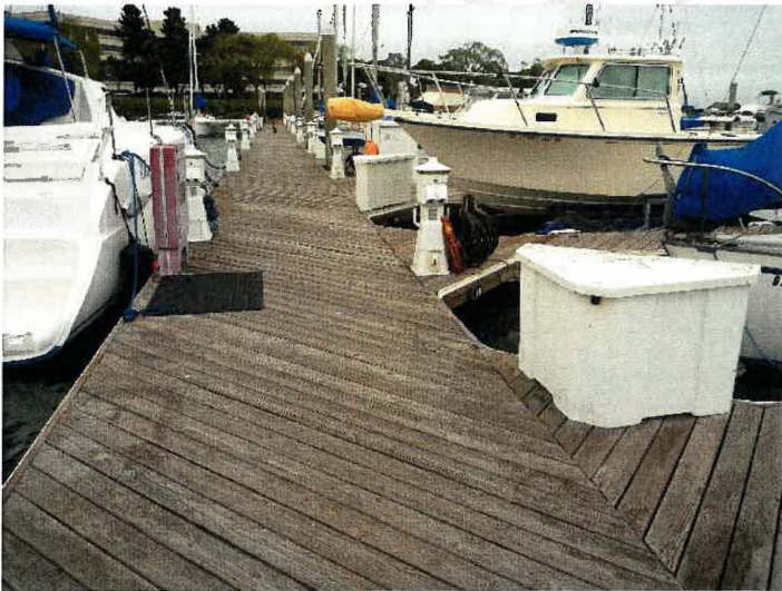
Photograph 1 General appearance of Docks 1 through 6
