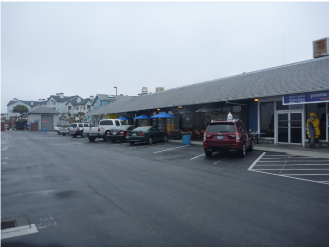
PHOTOGRAPH 8: TENANT ROW & PARKING
