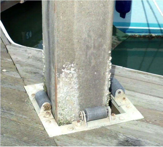
PHOTOGRAPH 1: TYPICAL PILE GUIDE -GOOD CONDITION (DOCK)
