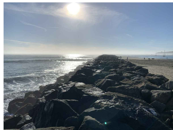
B EAST BREAKWATER - LOOKING WEST PHOTO
