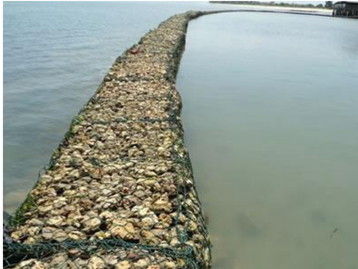
Figure 28 Gabion cages forming a breakwater
