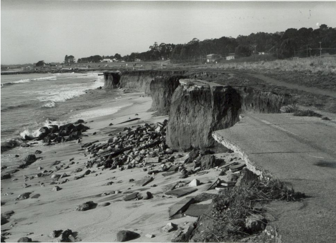
Figure 9 Photograph showing erosion of the Surfer's Beach shore looking north toward Pillar Point Harbor in 1971
