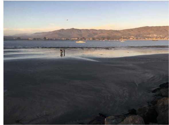
C WEST BREAKWATER - LOOKING NORTH EAST PHOTO
