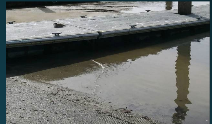
Launch Ramp Dredging Appropriation offset by FEMA
