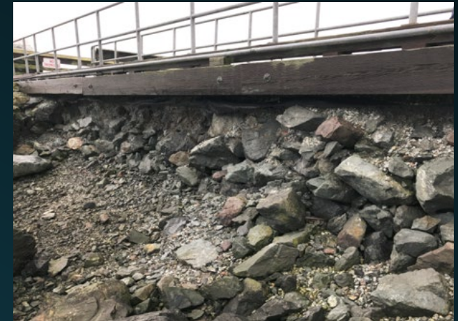
Fishing Pier Repair
