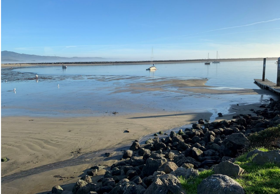
Figure 3: Photograph showing significant accumulation of sand near boat launch ramp in foreground and along the East Breakwater in background (1/13/21)
