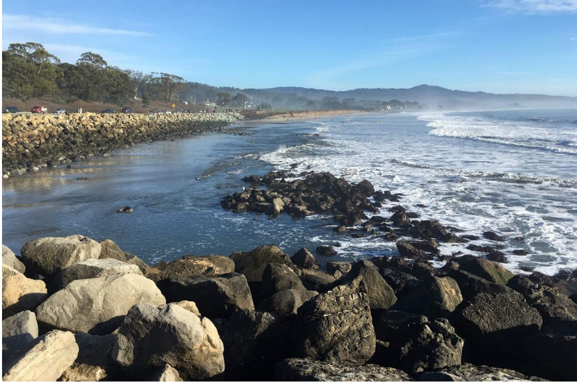
Figure 2: Photo of Surfers Beach on January 13, 2021 at low tide, showing Highway 1 at left with rock revetment, eroded beach and exposed rocks
