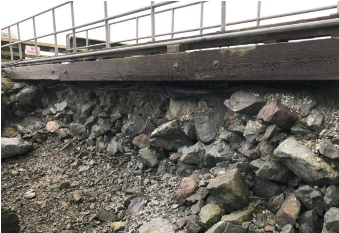
Along with the supporting rip rap erosion and failing timber issues, the Fishing Pier walkway and terminus platform need alteration for ADA compliance.
