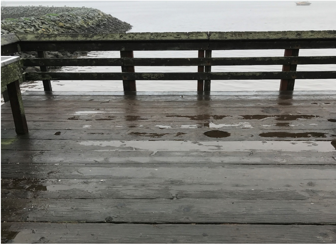
Along with the supporting rip rap erosion and failing timber issues, the Fishing Pier walkway and terminus platform need alteration for ADA compliance.
