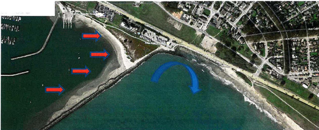
Figure 1. Sand buildup in Pillar Point Harbor (red arrows) and erosion at Surfer's Beach (blue arrow).
