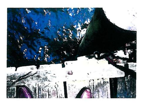
FENDER PILE BROKEN AT WATERLINE PHOTOGRAPH NO. 8
