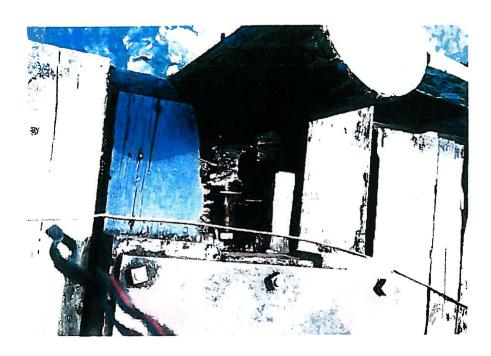
FENDER PILE CONENCTION DAMAGE AT DECK LEVEL PHOTOGRAPH NO. 7
