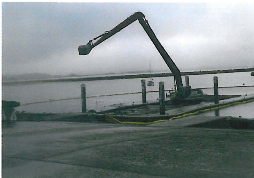
Figure 4 Offloading Material at Boat Ramp with Containment Boom
