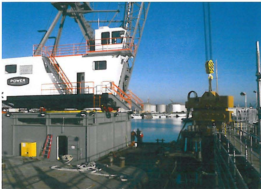
Figure 3 Barge Mounted Crane and Vibratory Hammer
