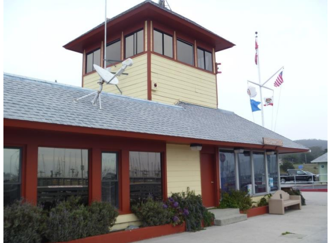
Photograph 4: Harbor Office Building
