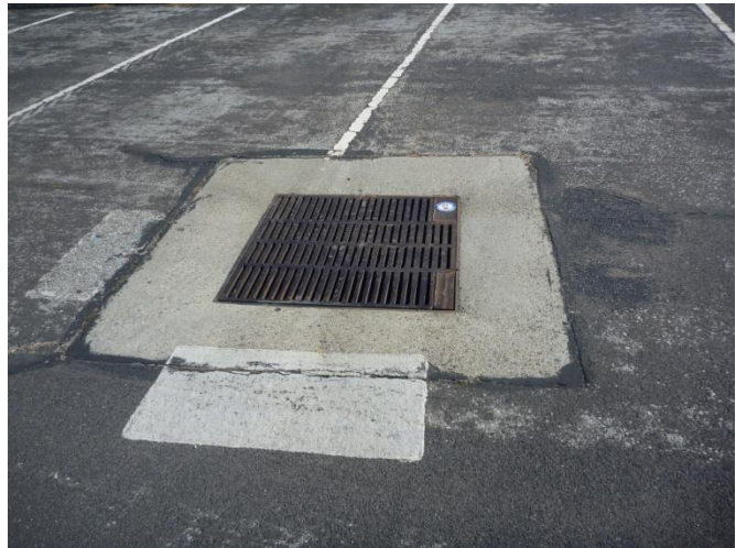
Photograph 15: Storm Drain Drop Inlet
