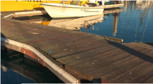
Johnson Pier H-Dock Replacement
