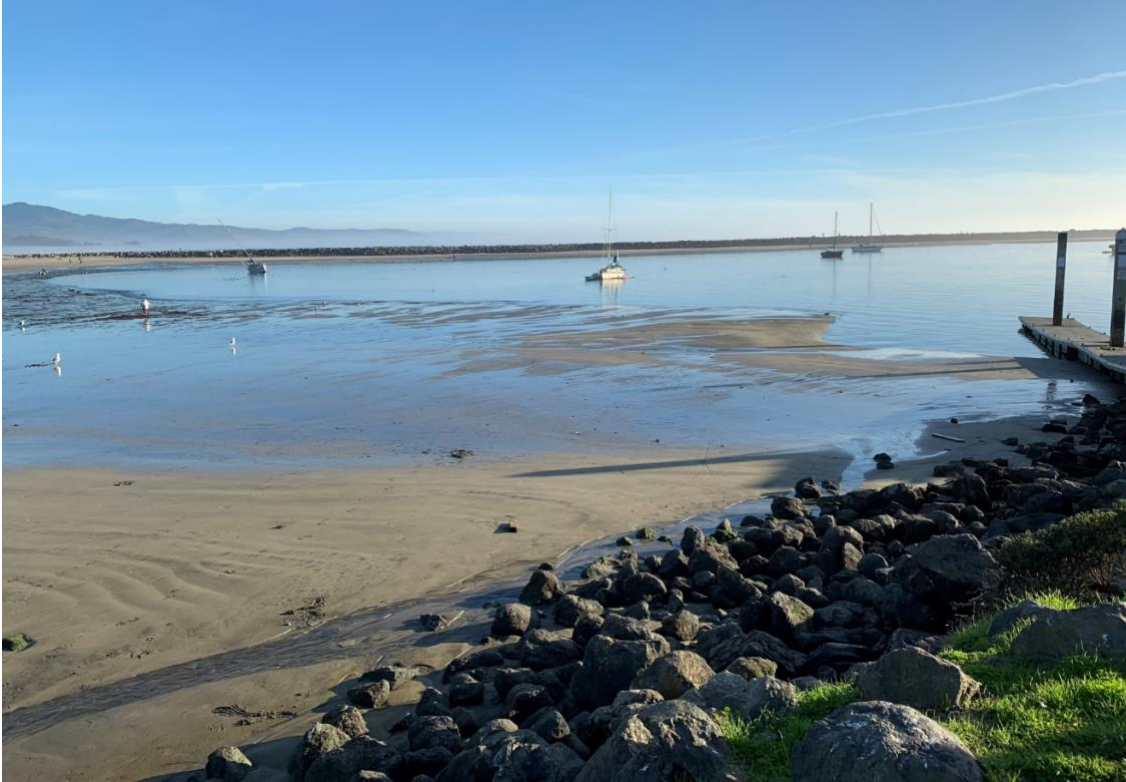
Figure 3: Photograph showing significant accumulation of sand near boat launch ramp in foreground and along the East Breakwater in background (1/13/21)
