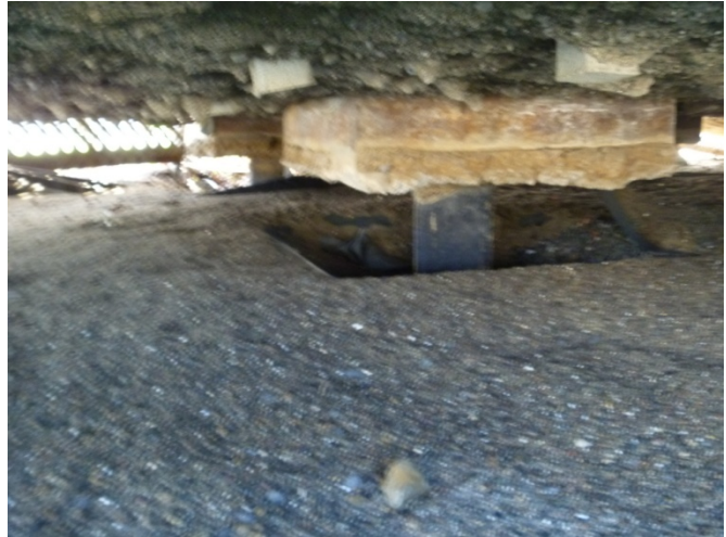
PHOTOGRAPH 3: HARBOR MASTER'S OFFICE BUILDING
