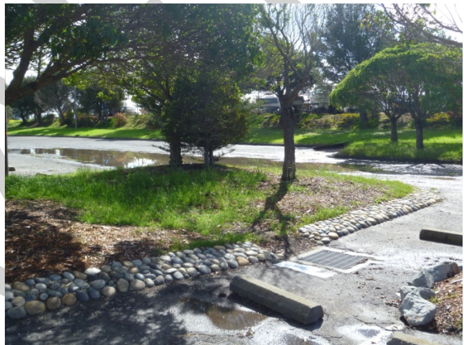
PHOTOGRAPH 14: STORM DRAIN AND STANDING WATER IN OYSTER POINT PARKING LOT
