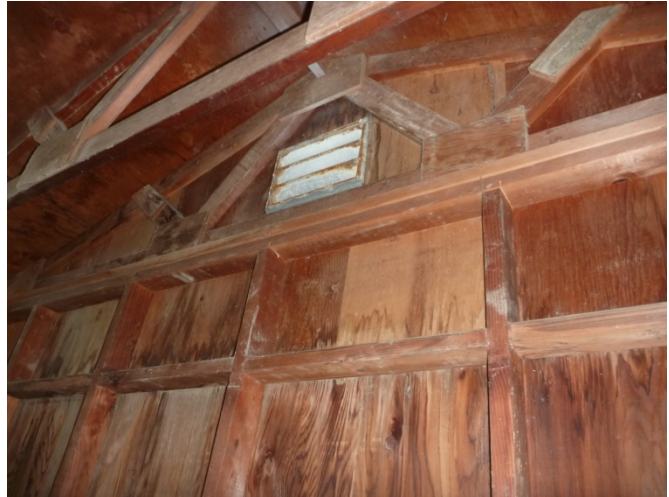
PHOTOGRAPH 8: ELECTRICAL VACUUM BUILDING
