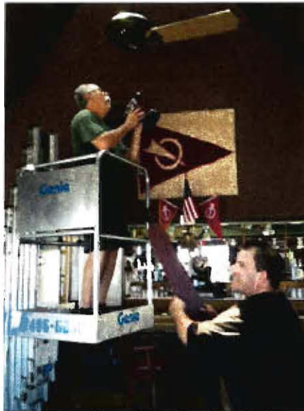
Disassembling the fan in the bar to clean above it
