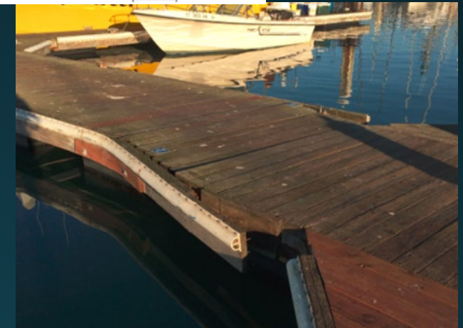
Johnson Pier Terminus, Fuel Dock Replacement & H-Dock Replacement
