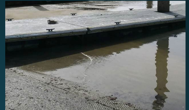
Launch Ramp Dredging
