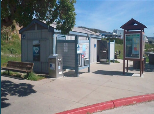
Launch Ramp Restroom/ Boat Wash/ Ramp Improvements
