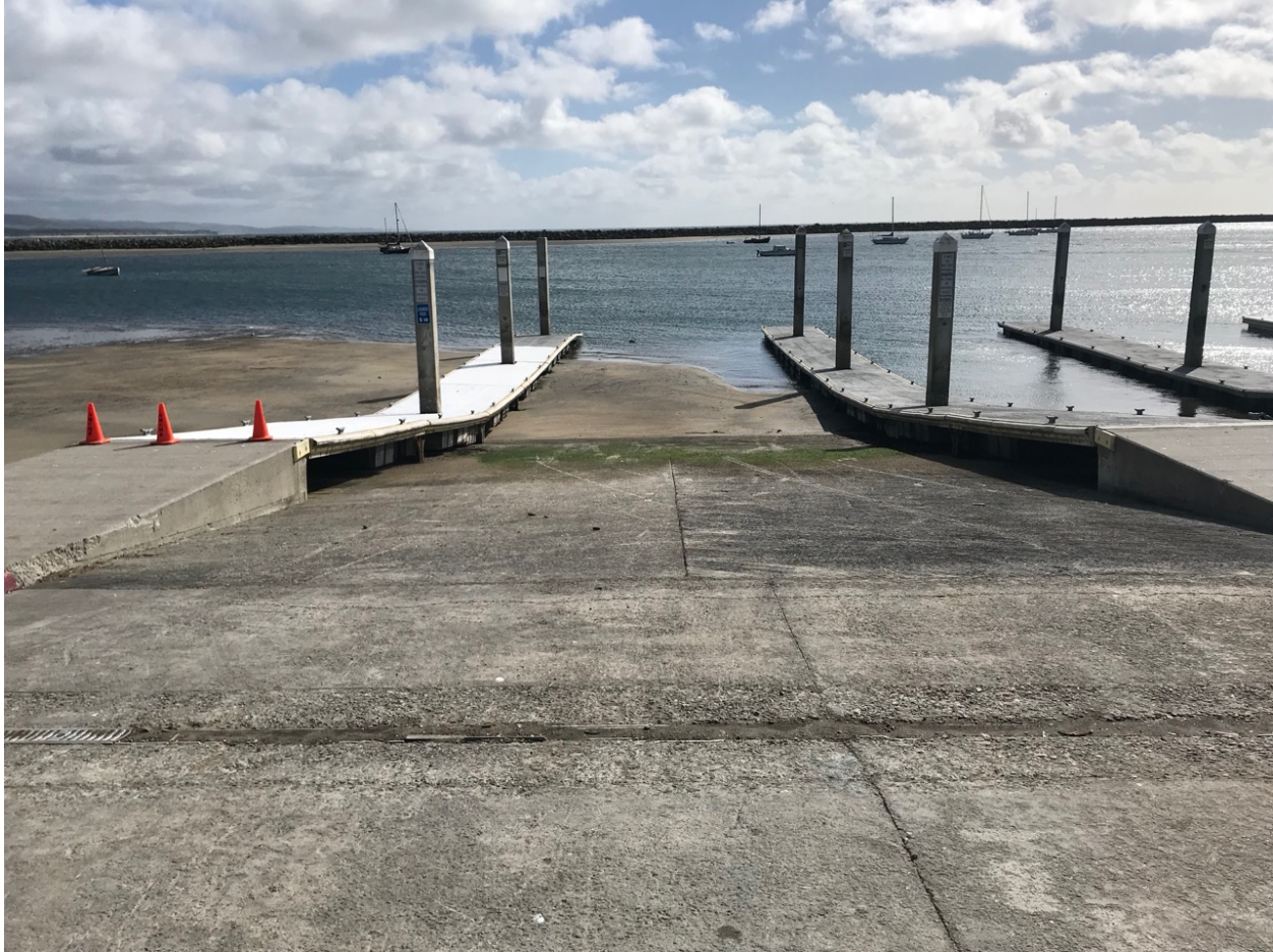
Photo showing shoaling at the PPH Boat Launch Facility
