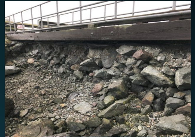
Fishing Pier Repair
