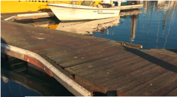
Johnson Pier H-Dock Replacement
